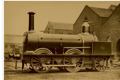
Beyer, Peacock and Company, Madras Railway (India) '0-4-2' tank locomotive Order No 425, 1860.
