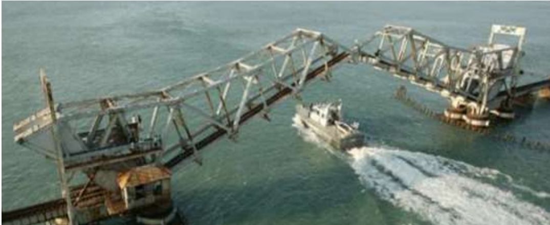
Figure 1: Photograph of Bascule section of Pamban bridge
